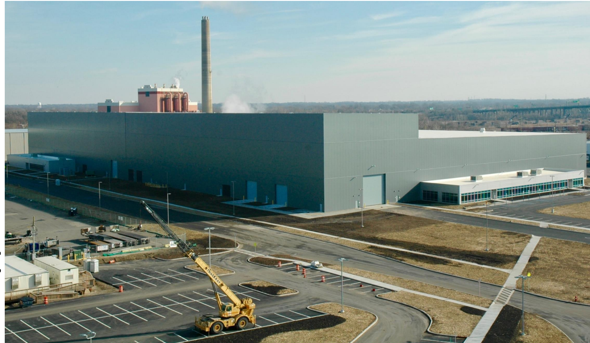
Holtec Advanced Manufacturing Division, Camden, NJ
