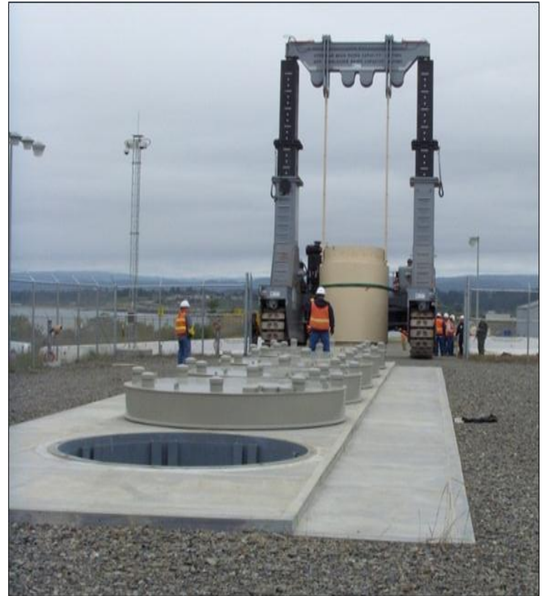
Below-grade Storage at Humboldt Bay Power Plant, Eureka, CA
