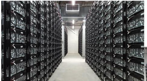
12,240 Li-ion Batteries1020 Battery Racks10 Inverters
