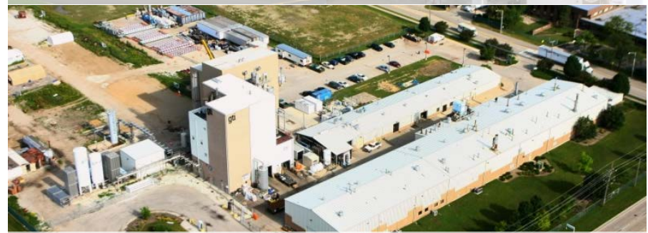
Energy & Environmental Technology Center
