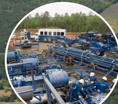
Completion/ Fracturing Operations
