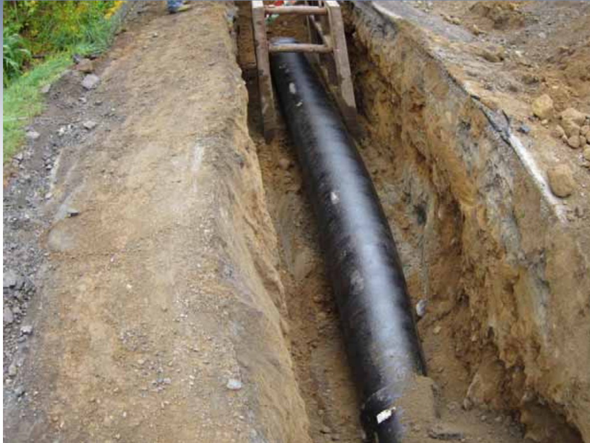
Water Main Installed
